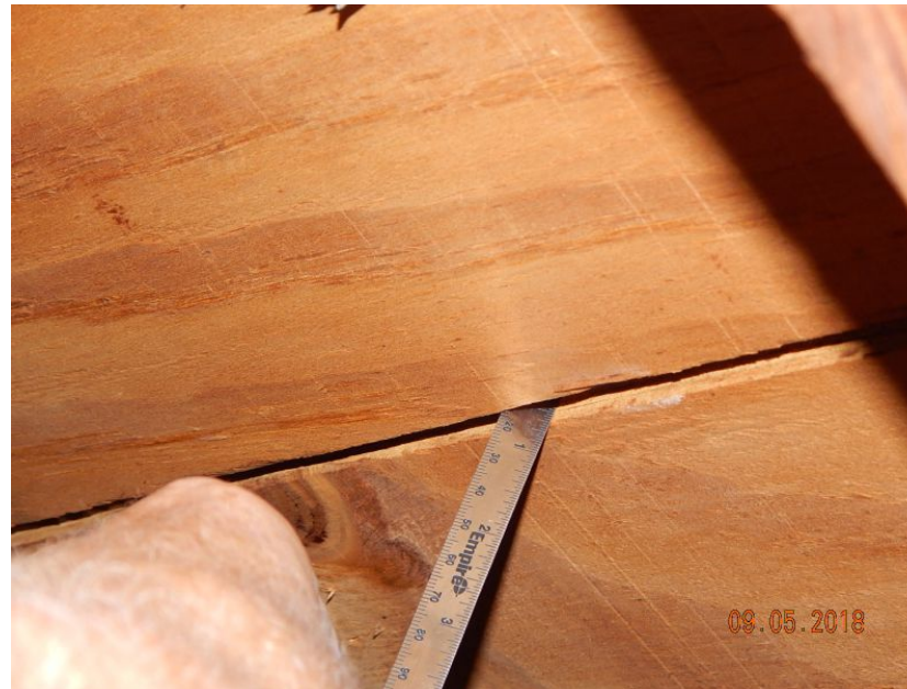
1/2" Deck Thickness Confirmed
