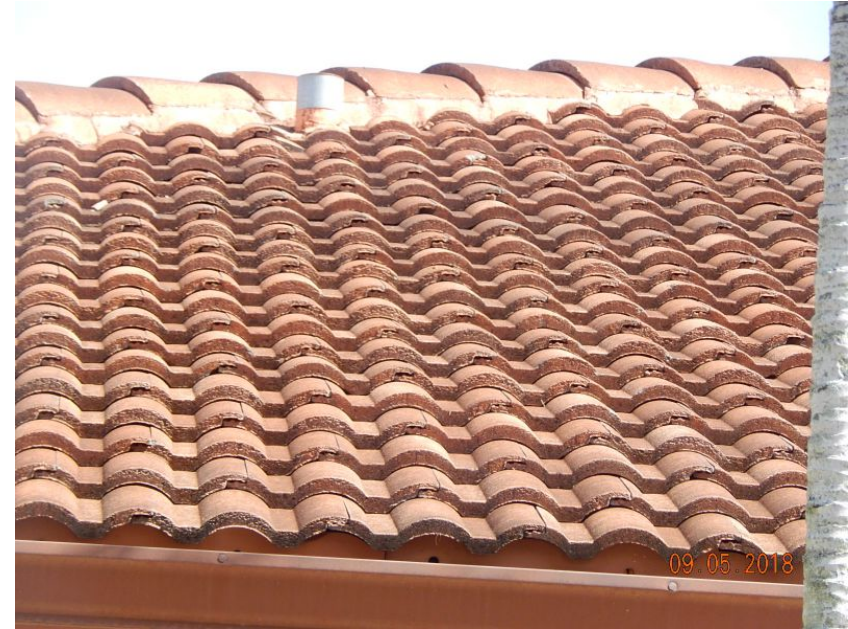
Concrete/Clay Tile Roof Covering
